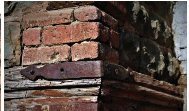
Piece of iron support at the corner of the wooden base, which was used to prevent the imbalance caused by huge load. Even after 150 years it is perfectly doing its job.
