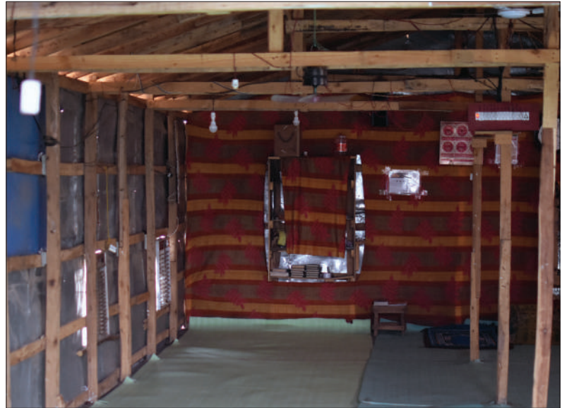
Interior of one of the sheds in the camp. The refugees have to pay Rs 1,000 as monthly rental charges. They spread rags on the ground to sleep. The sheds are mainly built of wooden poles and old steel sheets, while roofs are formed of foam sheets.
