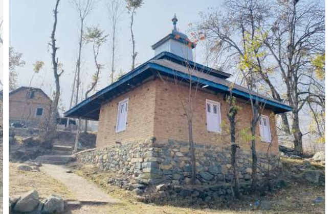
This mosque survived the avalanche at Waltengu Nar.
