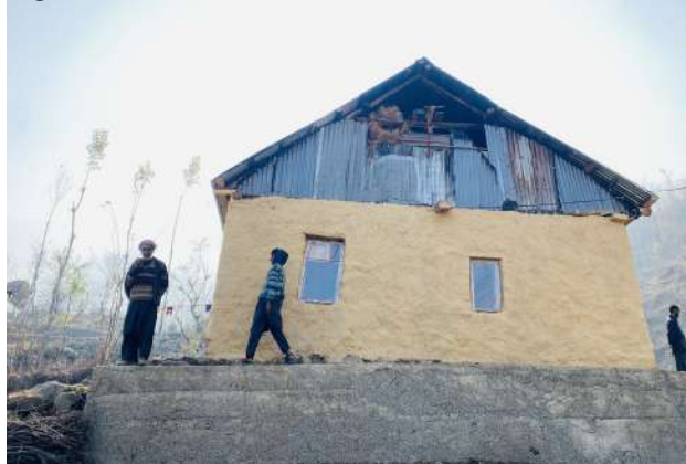
This house has been rebuilt by a victim post avalanche.
