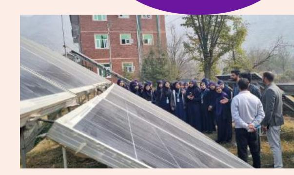
Solar photo voltaic on grid 2 KWP power mono Dual MPPT based technology DEPTT.OF Electrical Engineering IUST Awantipora
